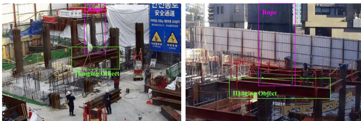
Fig. 4. Example images where hanging objects and ropes are not clearly visible due to complex background. (Images by authors.)
