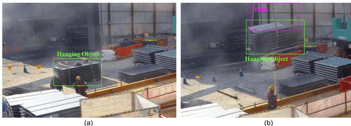
Fig. 3. Example images illustrating object shape invariance: (a) object on ground; and (b) object hanging from rope. (Images by authors.)
